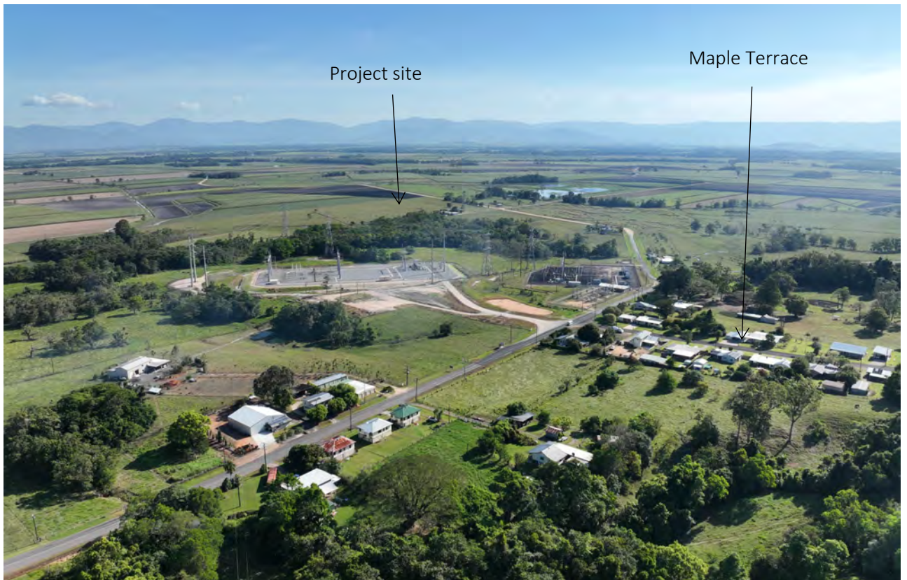
FIGURE 4-8: AERIAL VIEW OVER TULLY GORGE ROAD TO THE EXISTING AND UNDER CONSTRUCTION SUBSTATION
