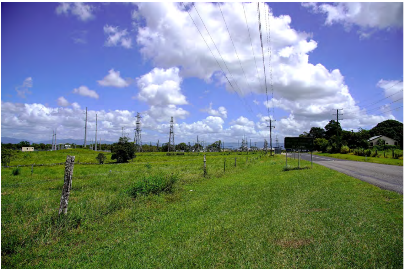
FIGURE 4-5 VIEW ALONG TULLY GORGE ROAD TO EXISTING TRANSMISSION LINES CONVERGING ON THE TULLY SUBSTATION
