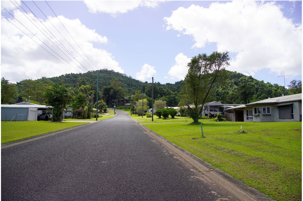
FIGURE 4-7: VIEW ALONG MAPLE TERRACE FROM INTERSECTION WITH TULLY GORGE ROAD
