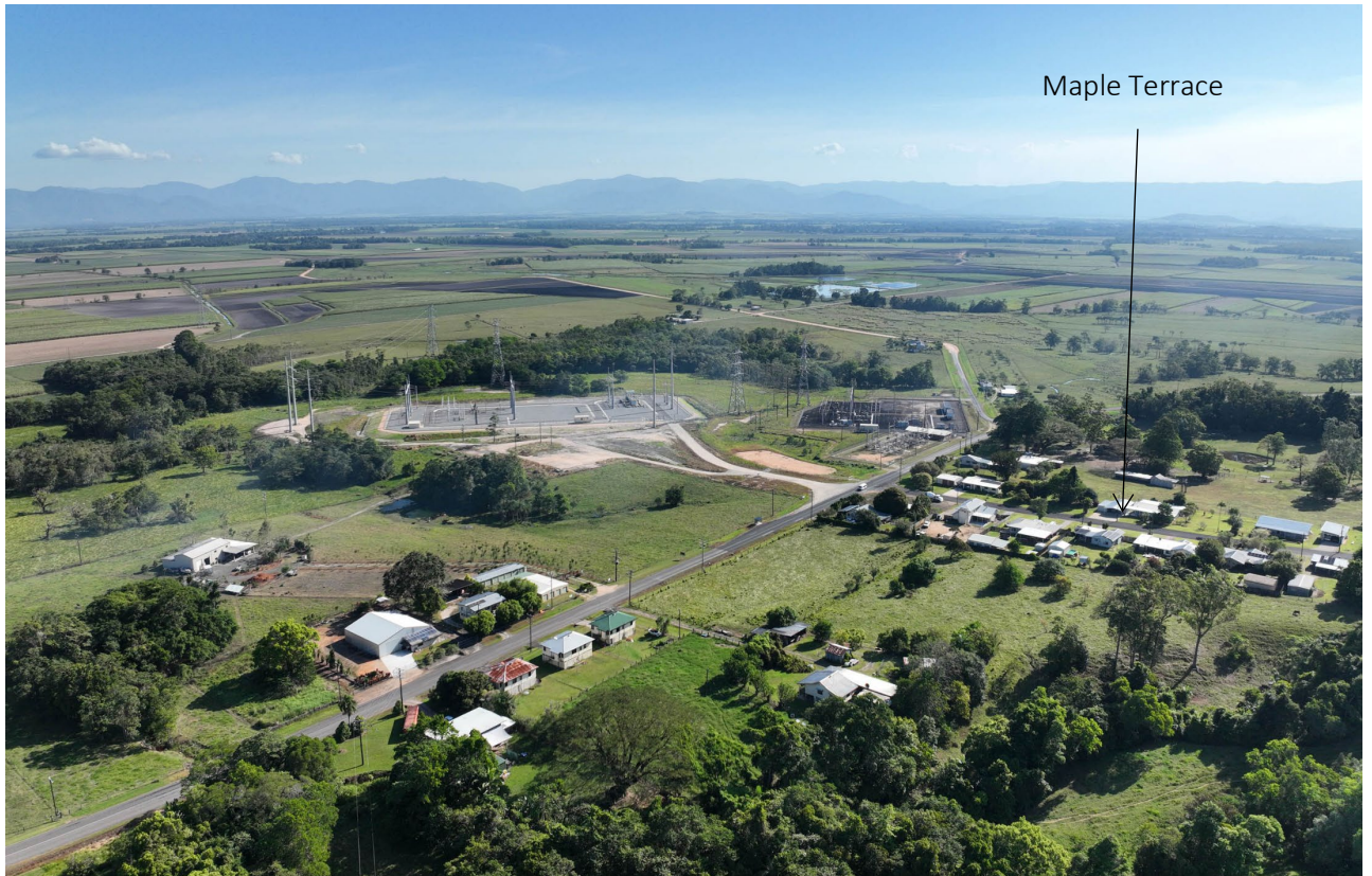
FIGURE 4-9: AERIAL VIEW OVER TULLY GORGE ROAD TO THE EXISTING AND UNDER CONSTRUCTION SUBSTATION
