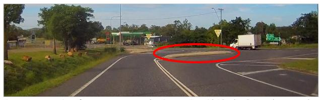
Figure 4.18 Street view of Dawson Hwy approach to intersection with island and sign to be removed
