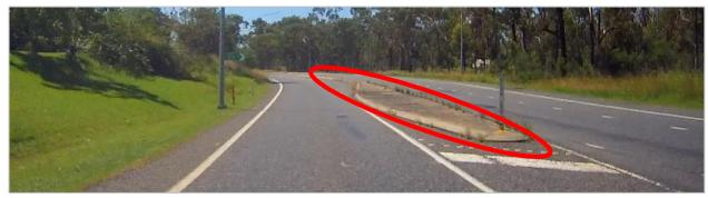
Figure 4.4 Street View of centre island to be removed from southern approach to intersection
