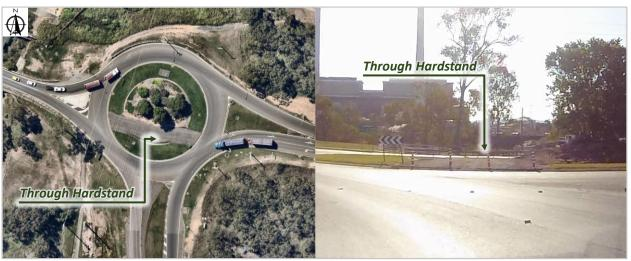
Figure 2.6 Hardstand added through Hanson Road / Red Rover Road roundabout for through movements.
