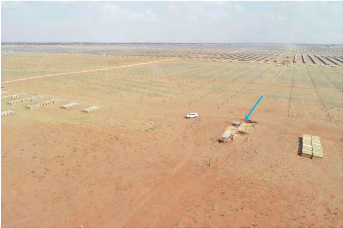
Plate B.1 Aerial view of the sun farm with the proposed location of the high voltage power station as indicated by the blue arrow. View south-east.
