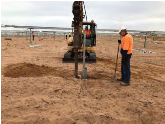
Plate 2.5 Example of post removal; view east
