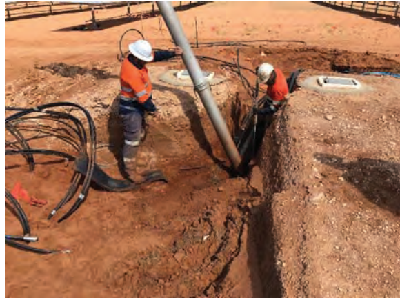
Plate 2.8 Monitoring sand removal within the isolator trenches in Block 84; view south
