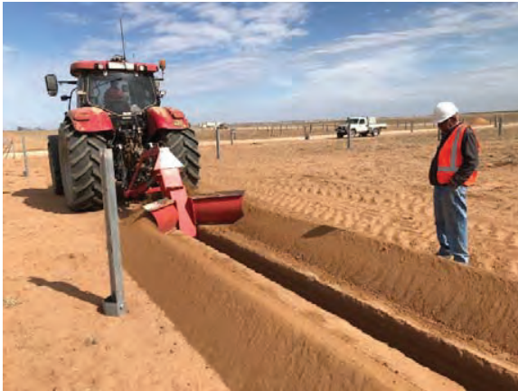
Plate 2.7 Monitoring trenching activities; view north-west
